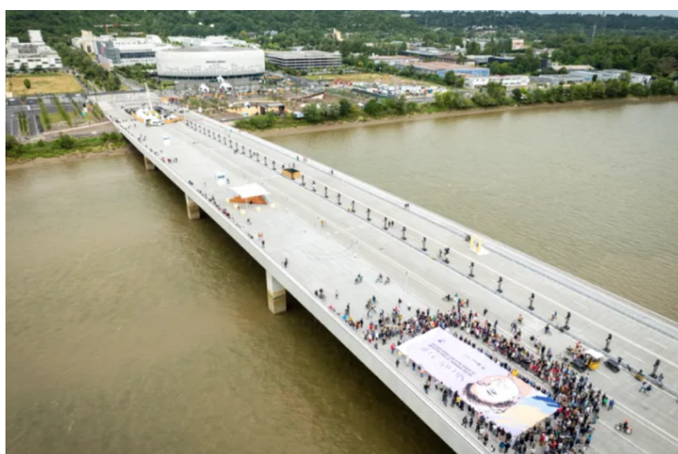
Obr. 63: Most Simone Veil, autor OMA/Rem Koolhaas a Chris van Duijn, Bordeaux, Francúzsko, 2024. Zdroj: [online] https://www.oma.com/news/simone-veil-bridge-designed-by-oma-rem-koolhaas-and-chris-van-duijn-opens-in-bordeaux .
