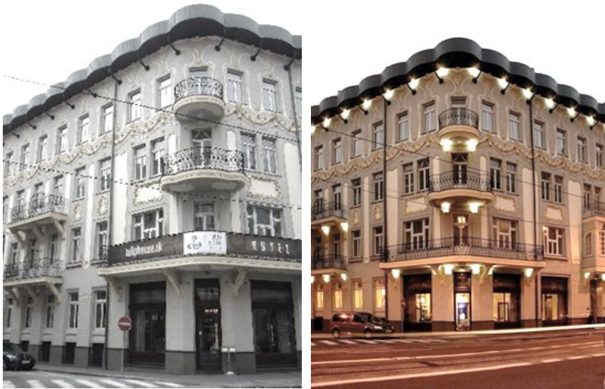
Obr. 55, 56: Roset Hotel & Residence, Bratislava. Zdroj: http://www.4-construction.com/sk/clanok/tulip-house-hotel-bratislava-zuzana-cambelova/
